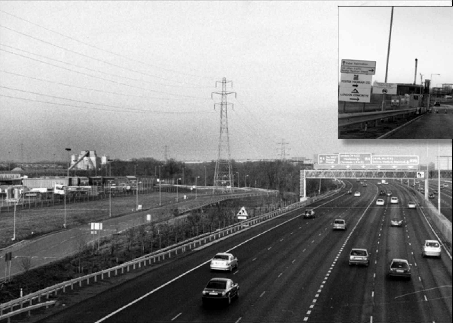
On the left London Concrete's plant in Heathrow can be seen from the motorway.
