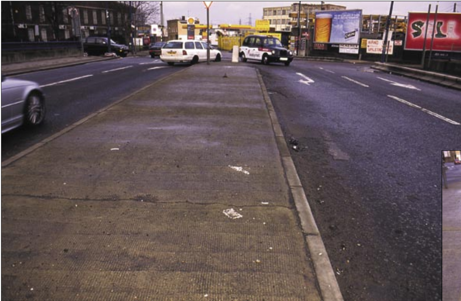
On the left Wick Lane above the A12, featuring visible spillage on the side of the road.
