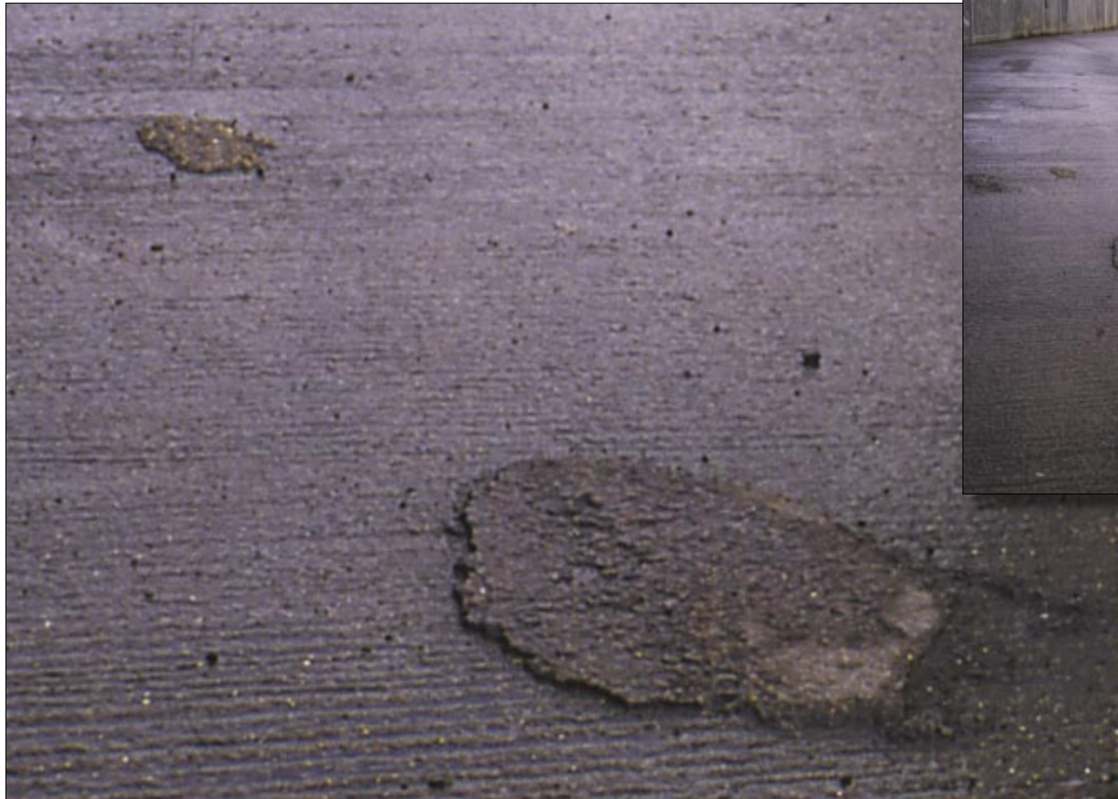
Bow | London Concrete entrance | 2 January 2006
