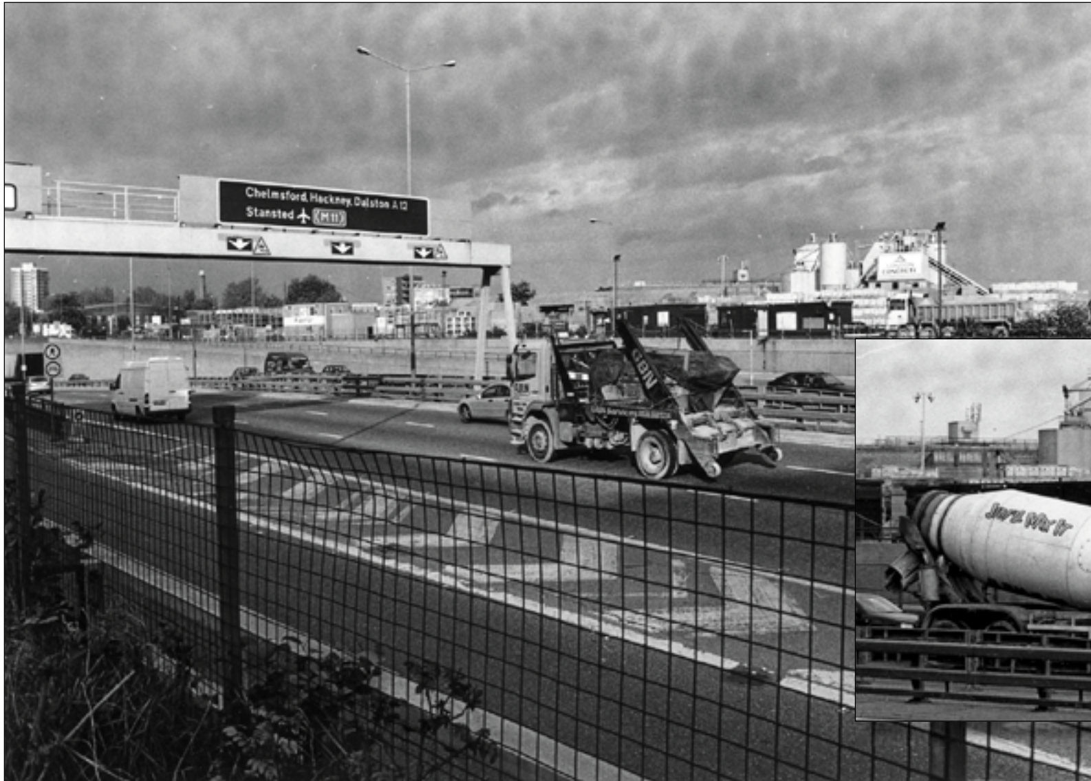
London Concrete batching plant in Bow viewed from the far side of the A12 showing full width of carriageway.
