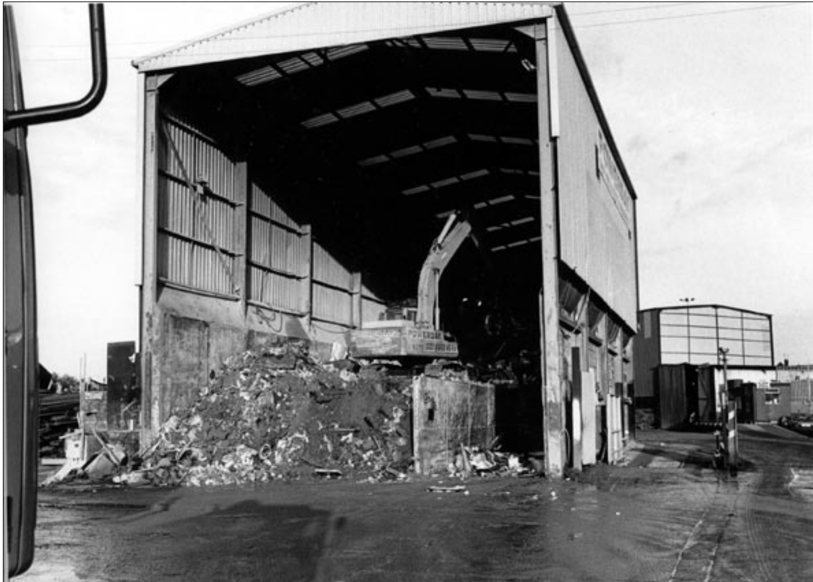
This picture shows the waste being processed by Powerday to the rear of London Concrete's site.
